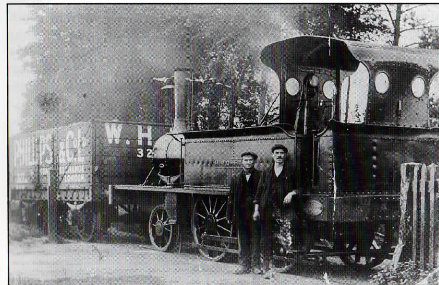
Brickyard Train - The Woolpit Brick & Tile Co. bought this Sharp Stewart 2-4-0 tank engine, Haro Haro to add to the 0-6-0 saddle tank engine which they already ran on the standard gauge line into the sidings at Elmswell. Haro Haro had previously seen service both on Jersey Railway and on the construction of the Manchester Ship Canal.
